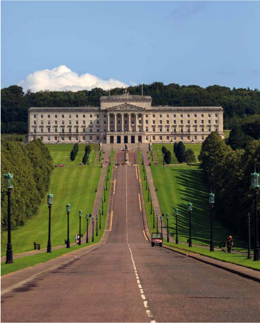
Figure 0.1. Stormont Building, Belfast, 2007. Purchased from iStock, image credited to VisionsbyAtlee.
